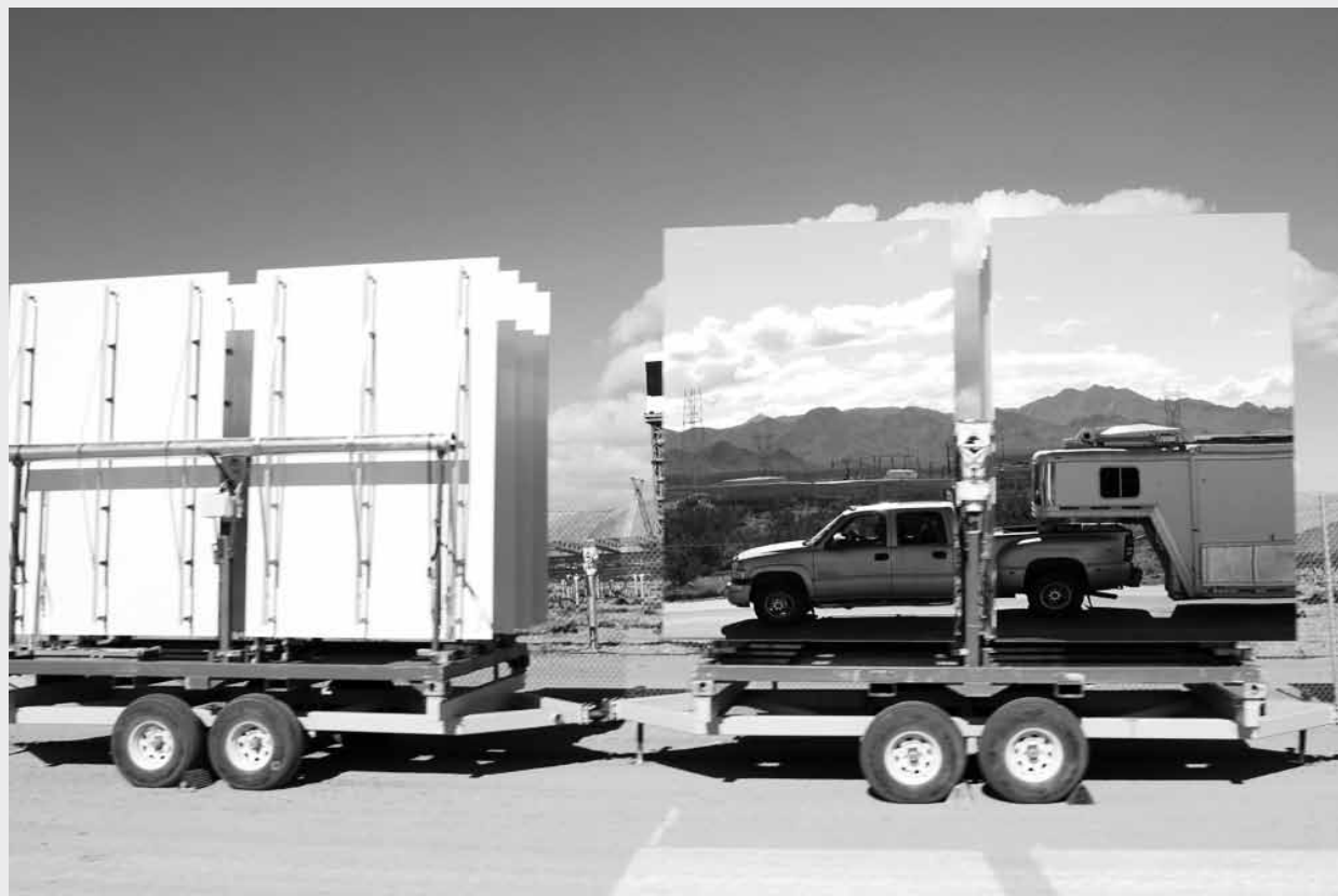
The Semester In the West truck and trailer drives past another trailer stacked with mirrors at the Ivanpah solar thermal power plant site in Southern California. Each mirror is part of a heliostat, a device that tracks the sun to reflect light and heat to a central “power tower” (the structure peeking out behind the mirror).
