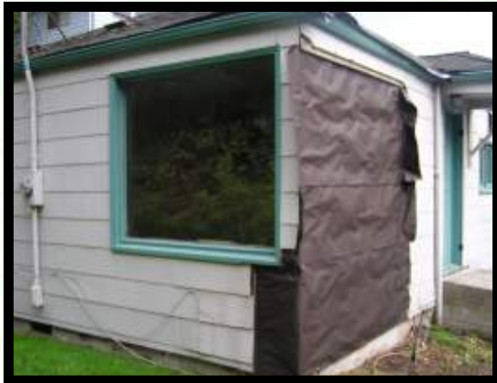
Asbestos "CAB" siding
